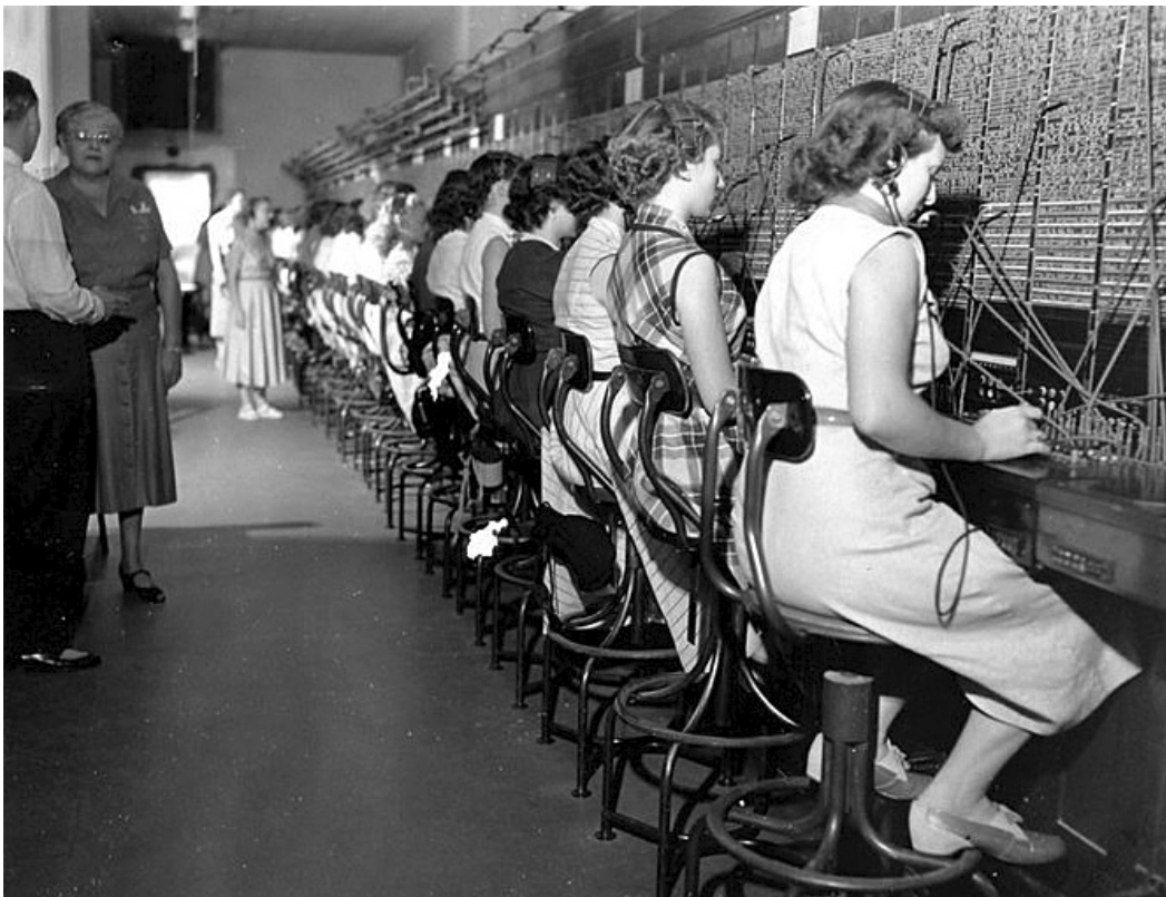
Figure 1. Typical manual switchboard lineup
