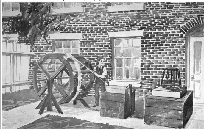
APPARATUS IN BACK YARD FOR PAINTING COTTON-COVERED COPPER WIRE E. T. HOLMES AT THE WHEEL—1862-64
