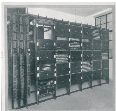
THE 300/500 "RELAY" AUTOMATIC TELEPHONE EXCHANGE WHICH SERVES BRITANNIC HOUSE, LONDON. THE OFFICES OF THE ANGLO-PERSIAN OIL COMPANY.
